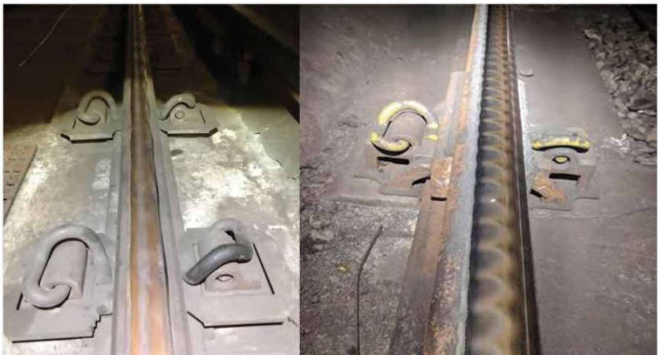
Figure 7: Short wavelength corrugation on LUL
